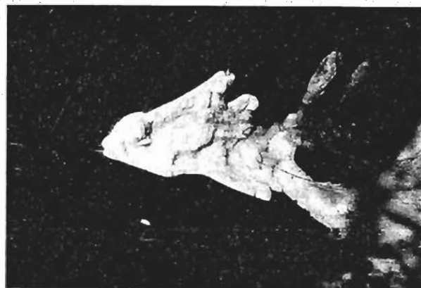
Early reproductive growth in the form of thickened, white and localised structure forming, in this case, at the junction of floorboards and joist
