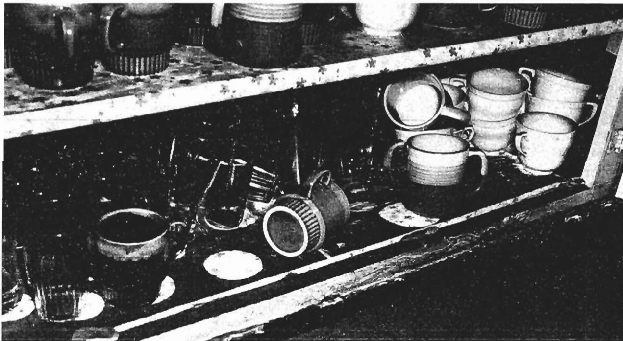
Deposit of billions of spores (coloured brick red) released by a mature fruit body located somewhere else in the building. The spores have settled on the horizontal shelving as shown by the area from which crockery has been moved immediately prior to photography
